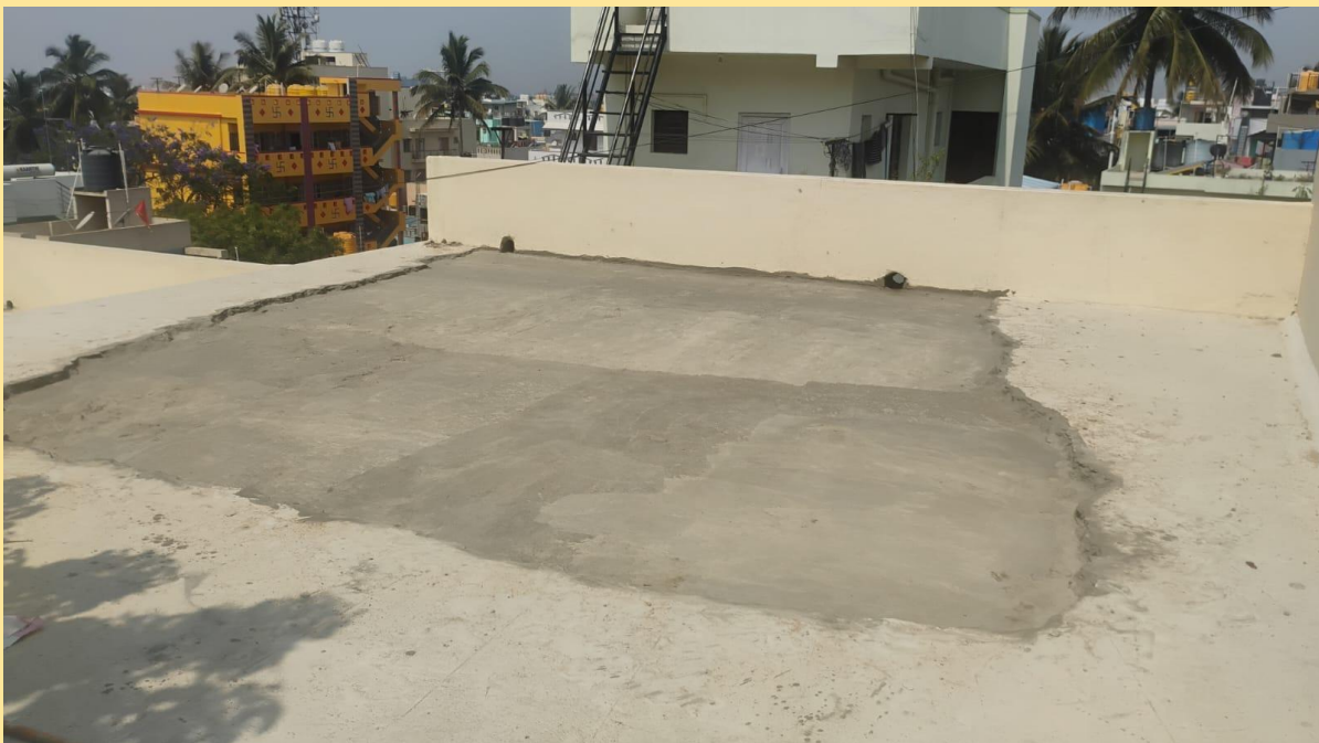
Terrace repair work completed to prevent water leakage
